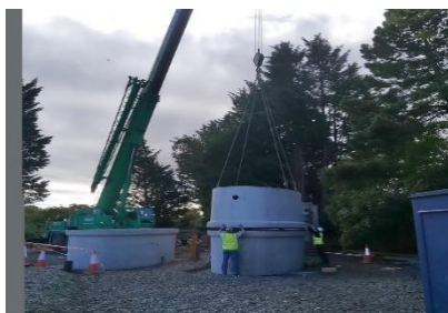
Installation of Settlement Tanks, Barndarrig.
